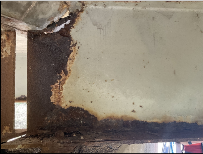
Span 2 bent 3 girder 4 6" x 1" hole @ haunch
