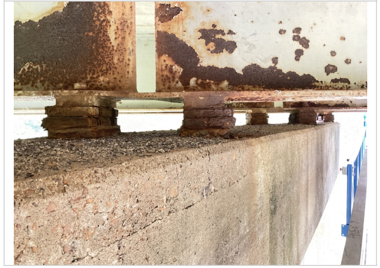
Typical bearing shims
