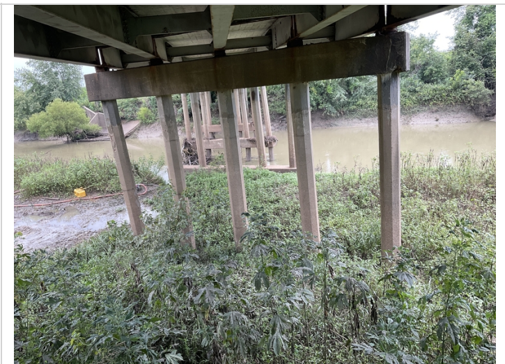
Piles out of plumb
