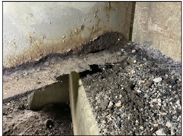
Span 1 bent 1 girder 4 - 8" x 1" hole at bottom of web 5" from end. 13" x 3" hole left bottom flange.
