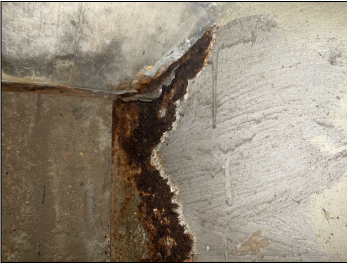
Span 7 bent 8 girder 4 10" x 1" hole @ haunch
