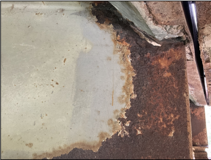
Span 6 bent 6 girder 4 6" x 1" hole @ haunch
