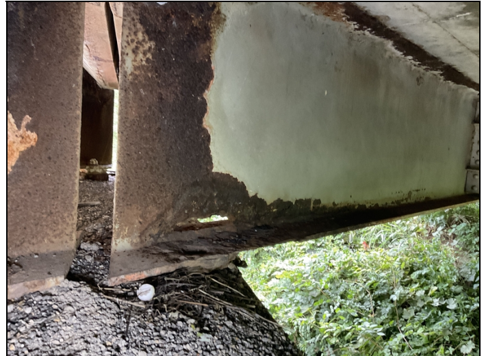
Span 1 bent 2 girder 4 9" x 2" hole @ bottom of web 6" from end. Knife edge bottom flange.
