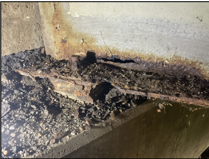
Span 1 bent 1 girder 4 3" x 2" hole right bottom flange
