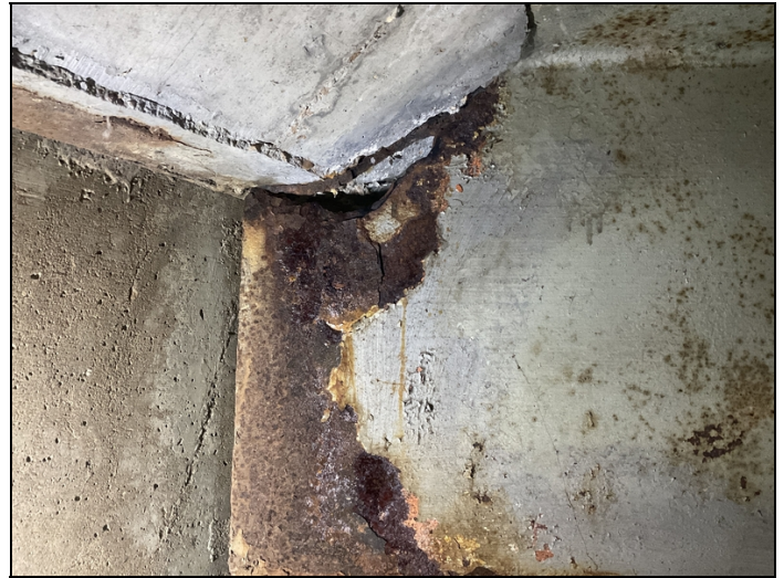
Span 1 bent 1 girder 2 9" x up to 2" hole @ haunch
