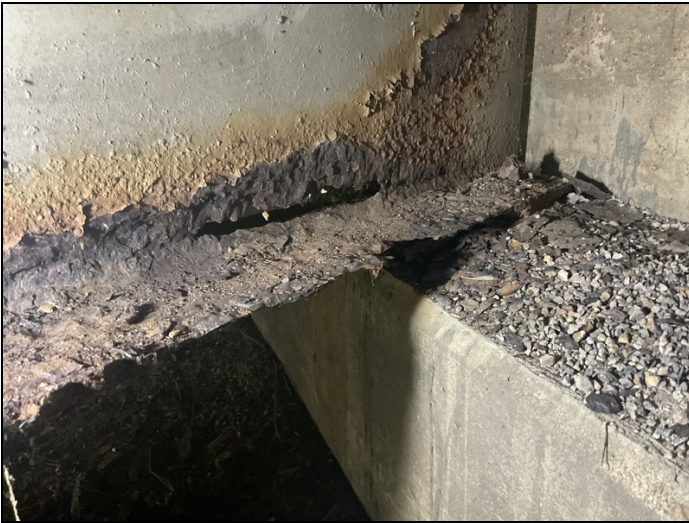
Span 7 bent 8 girder 3 Rt 18" x up to 1" hole in bottom of web 9" from end of girder, and a 4" x 2" hole in Rt bottom flange.
