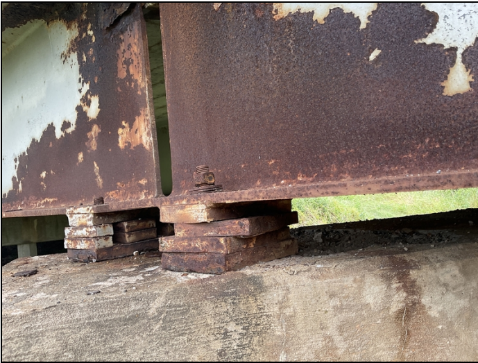
2023 - Span 5 bent 6 bearing 1 shims
