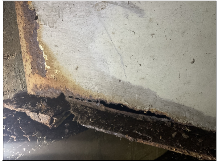
Span 7 bent 8 girder 3 Lt 18" x up to 1" hole in bottom of web 9" from end of girder, and a 6" x 3" hole in Lt bottom flange.
